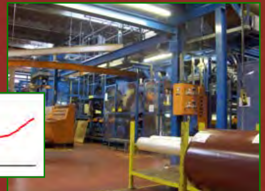
(21 section drive.web system on an embossing line)
